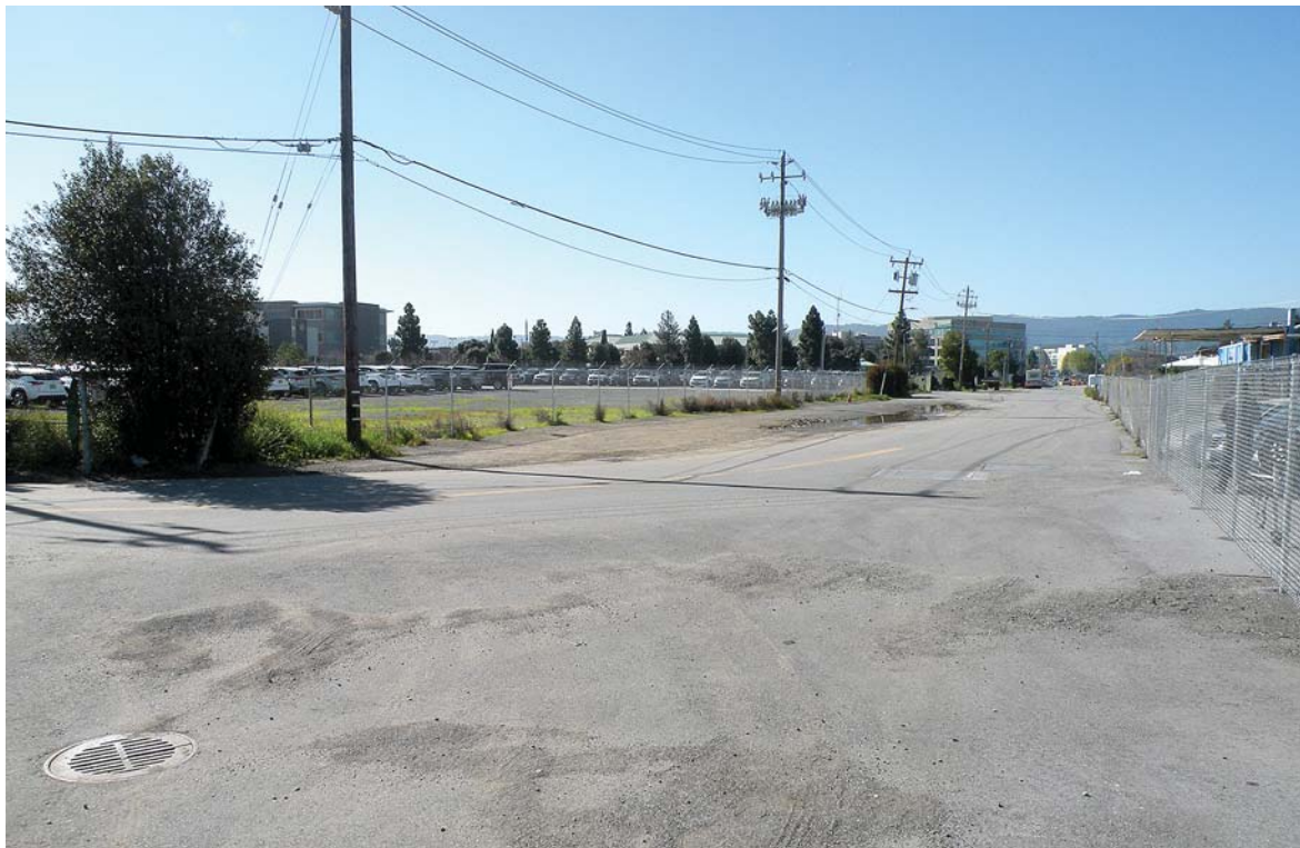
Photo 4: Surface Roadways and Parking Areas
