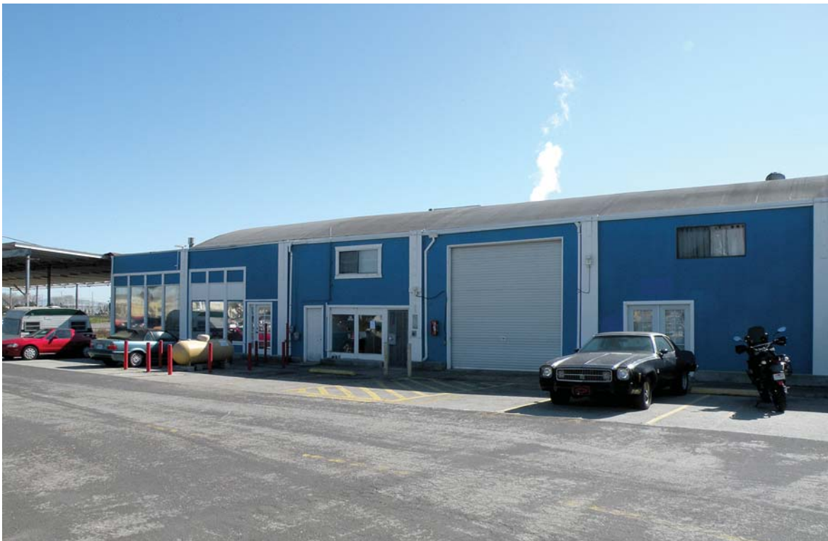
Photo 2: Existing Marina Maintenance Operations Building
