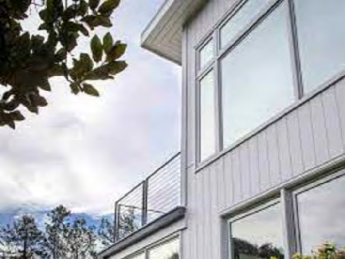
PANEL SIDING CREATING VERTICAL FACADE PATTERN WITH 6" AND 11" EXPOSURE
