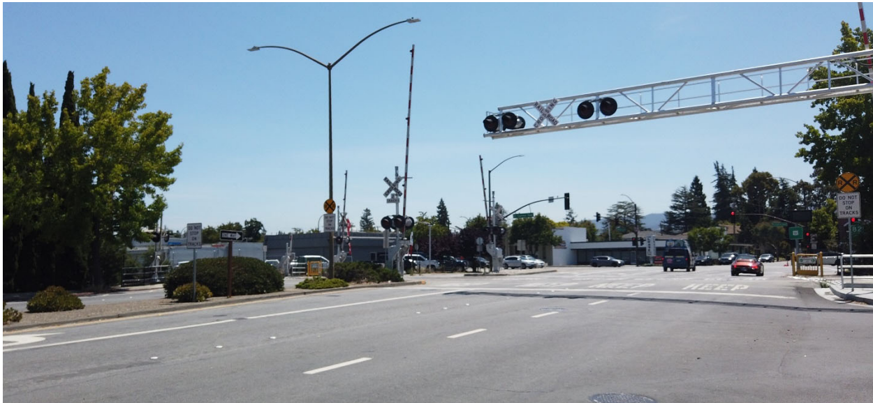
Photo 1: Whipple Avenue, Looking West from Stafford Street
