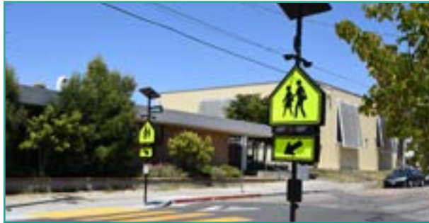
Rectangular Rapid Flash Beacon (aka Lighted Crosswalk)
